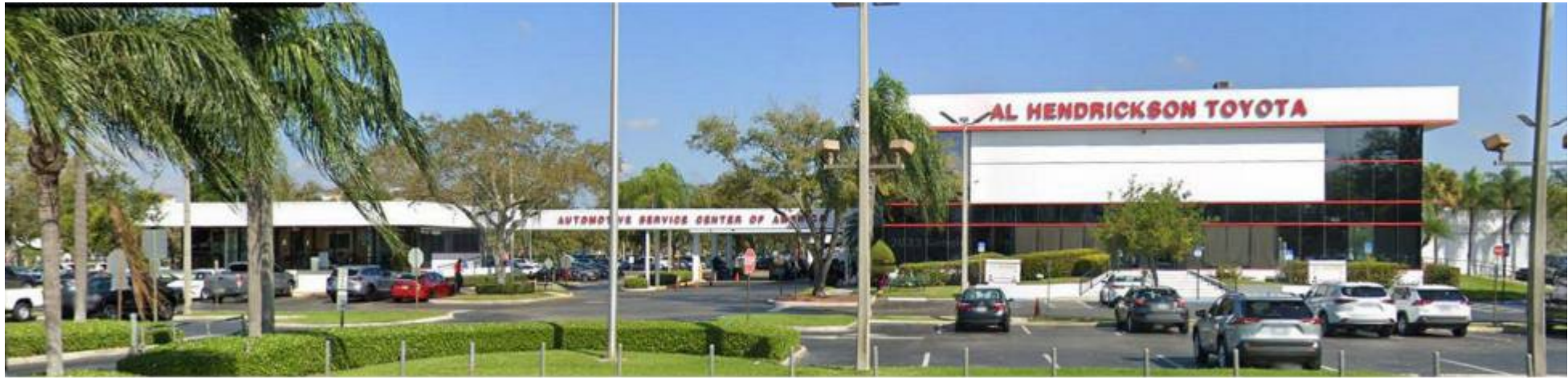
EXISTING FRONT VIEW
