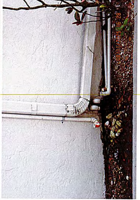
4753 NW 22 St ( Bayport II) observed a/c unit had been installed in closet with drainage outside instead of above the entry door on 8/11/25. JM
