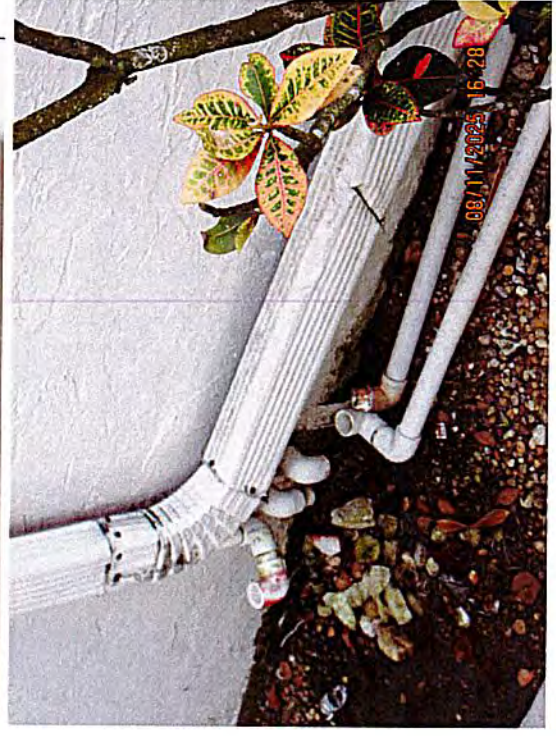
4753 NW 22 St ( Bayport II) observed a/c unit had been installed in closet with drainage outside instead of above the entry door on 8/11/25. JM
