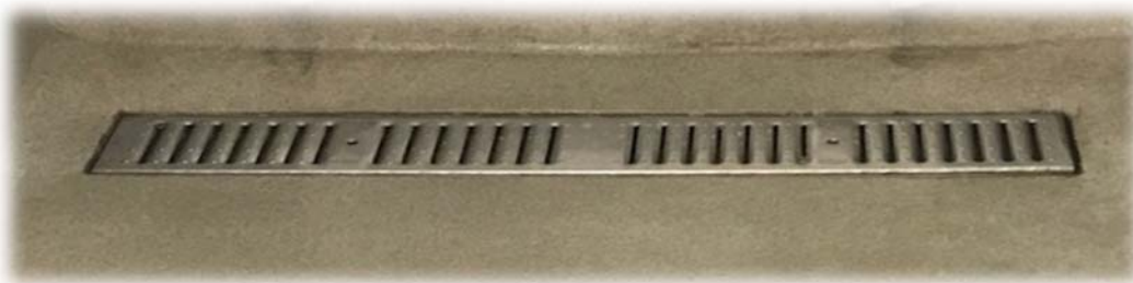
Figure 22 - Drain and Non-Porous Flooring in Each Kennel
