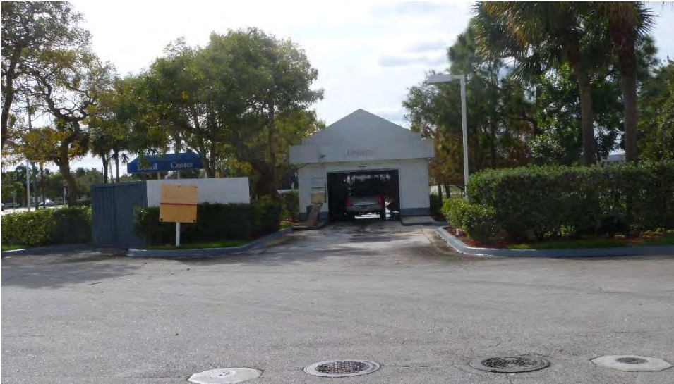
Car wash in operation (Looking West)
