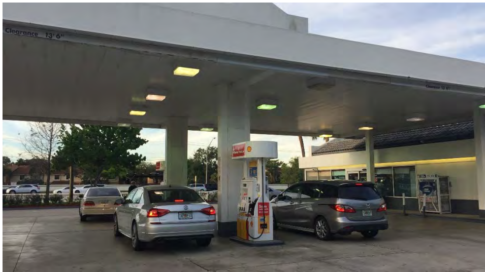
Gas pumps in operation east of convenience store (Looking South)
