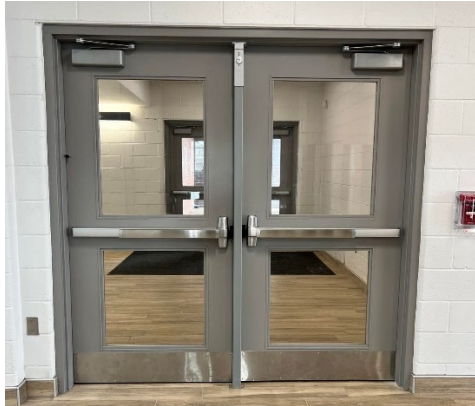
Flush mount panic hardware example
